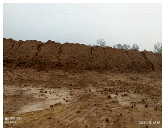
Picture 13: Constructional activities at site Toyontoli
