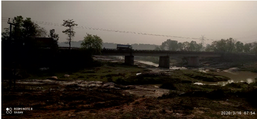
Picture 14: Bridge connecting the National Highway at site Toyontoli
